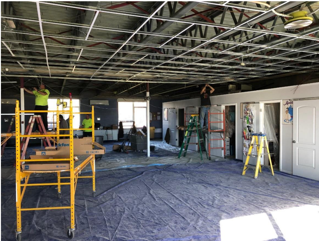
INSTALLING NEW CEILING IN MP ROOM – NOVEMBER/DECEMBER 2022
