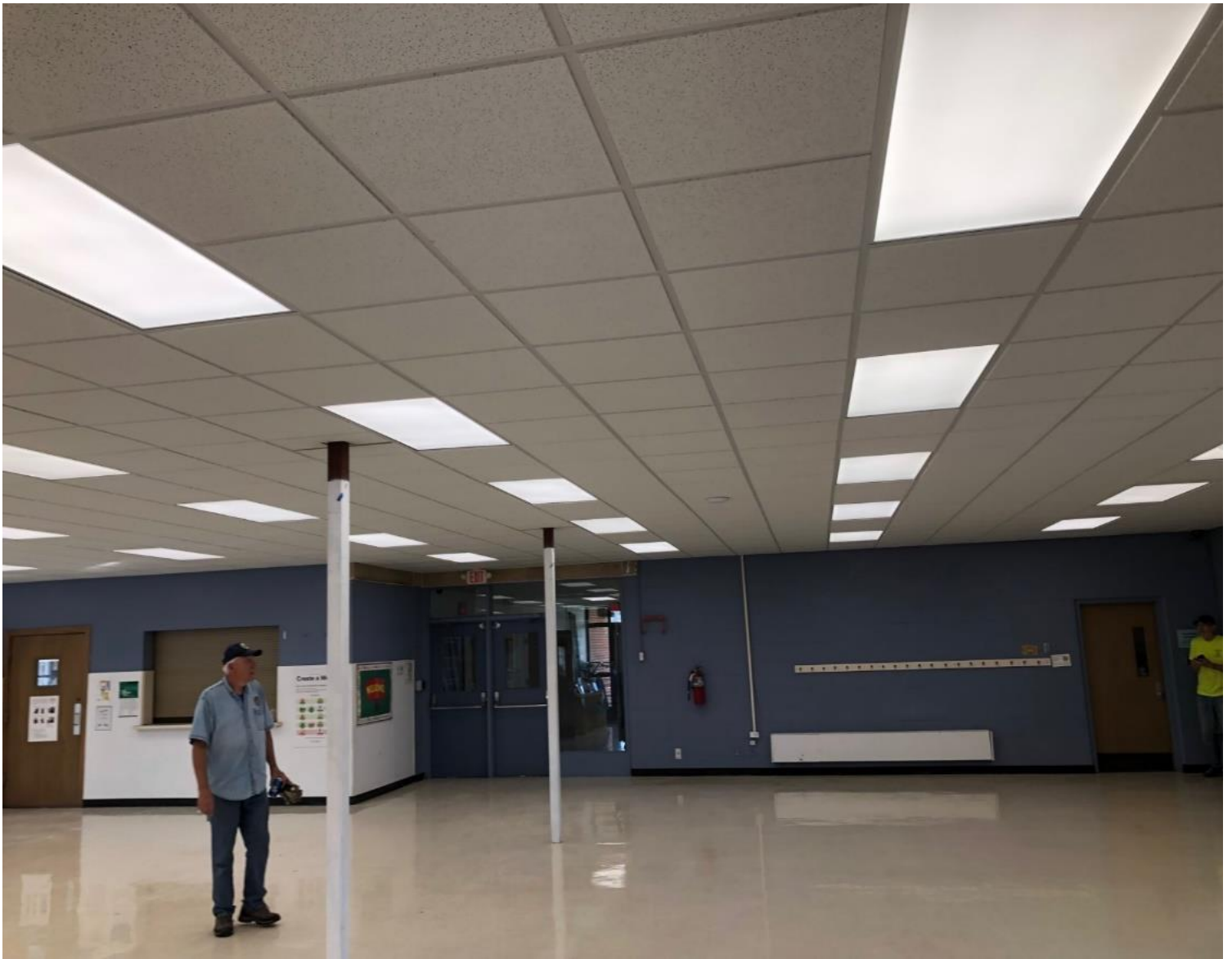
MP ROOM WITH NEW CEILING & OVERHEAD LIGHTS
