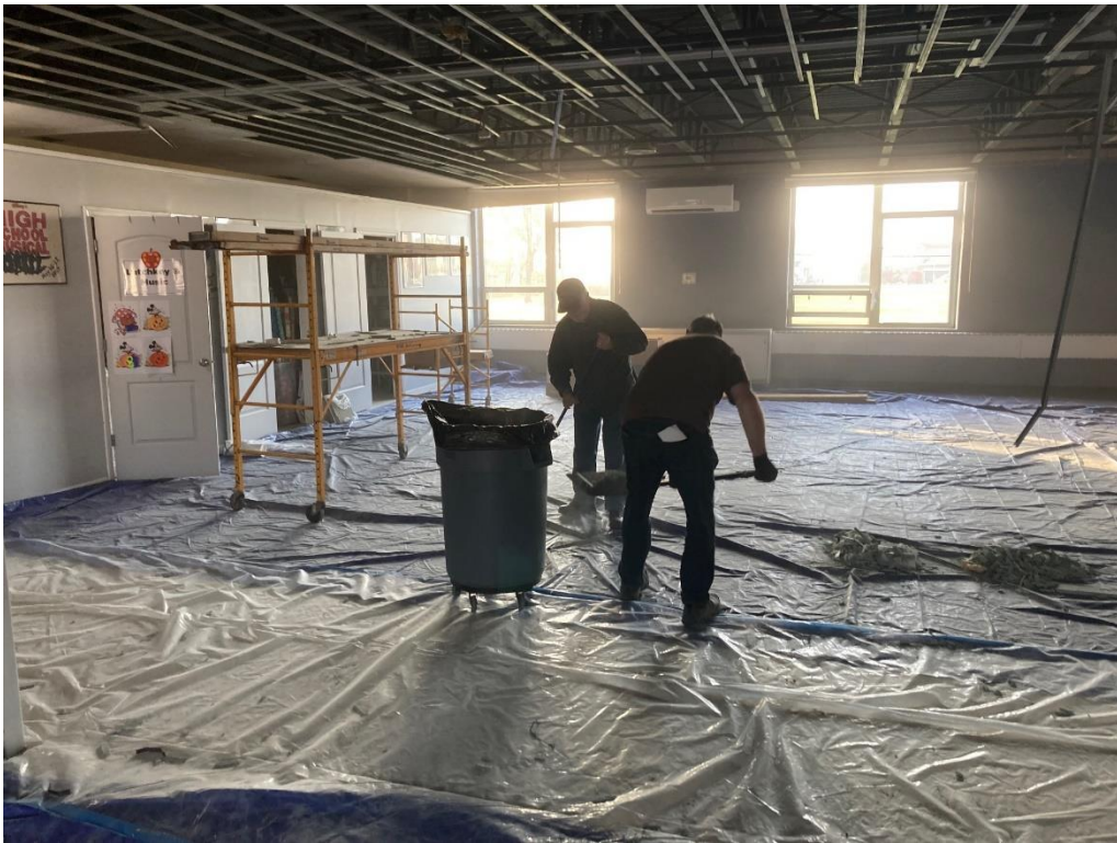
REMOVING EXISTING CEILING IN MP ROOM – NOVEMBER/DECEMBER 2022
