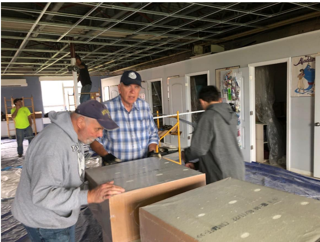
BROTHERS BOB & JIM GETTING MORE CEILING TILES
