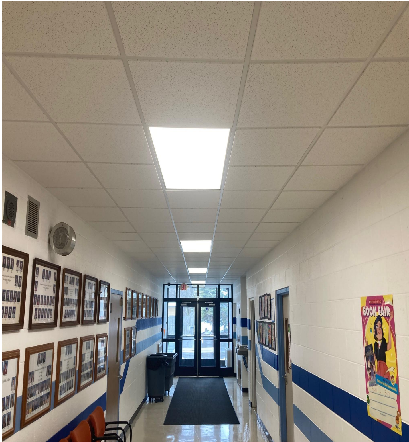
NEW CEILING IN HALLWAY – JUNE 2022
