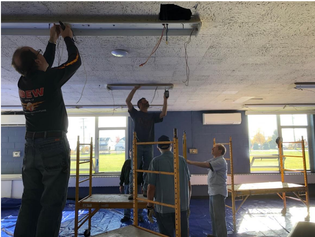
REMOVING EXISTING CEILING IN MP ROOM – NOVEMBER/DECEMBER 2022
