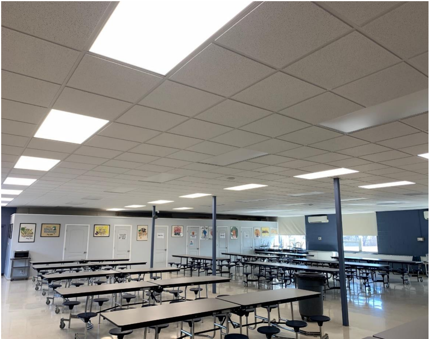
MP ROOM WITH NEW CEILING & OVERHEAD LIGHTS
