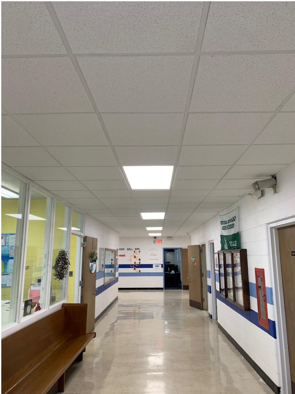
NEW CEILING IN HALLWAY – JUNE 2022
