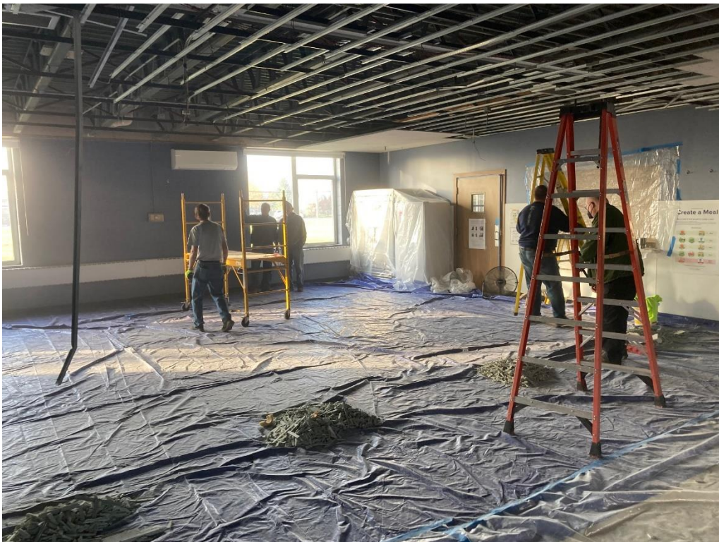
REMOVING EXISTING CEILING IN MP ROOM – NOVEMBER/DECEMBER 2022
