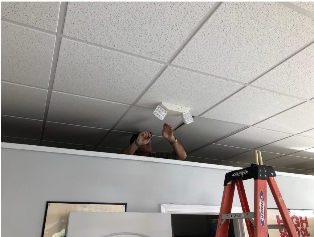
NEW EMERGENCY LIGHTS BEING INSTALLED
