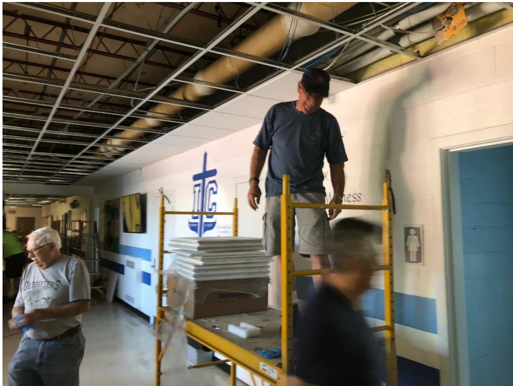
REMOVING EXISTING CEILING IN HALLWAYS – JUNE 2022
